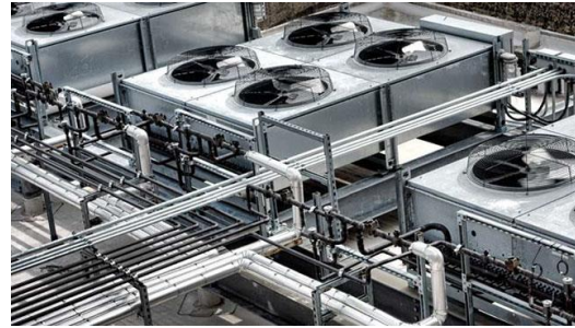
Figure 4: Outdoor Condenser Unit example.
